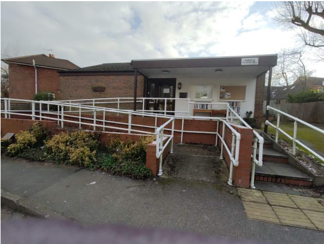
Fig 5: view of the village hall entrance and extensive ramps and steps
